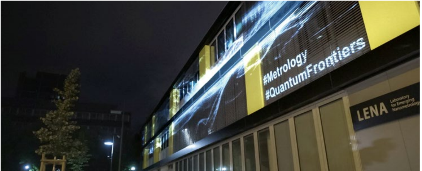
The new LENA building. © christo.cc/TU Braunschweig
