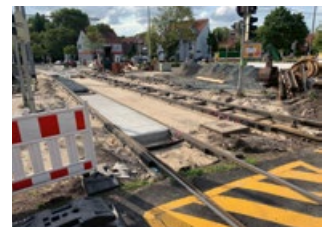
Construction side of public transport
